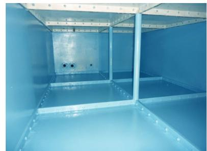
This special cold water tank lining system can be post cured in four hours, meeting all current regulations for drinking water.
