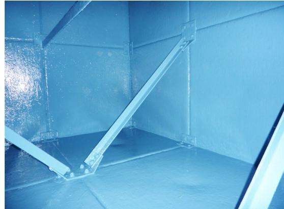
This is a surface tolerant tank lining system for use on all water tanks, cooling towers and air handling units.
